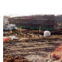
Locker North Wall - Valley Stadium
