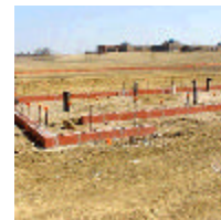
Restroom Block Walls - Valley Stadium
