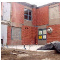
Northwest Addition Slab - Stilwell
