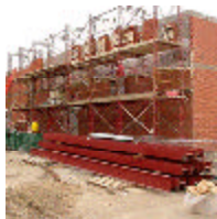
Mechanical Room Addition - Stilwell
