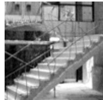
Stairway Demolition - Stilwell
