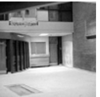
Stairway Removed - Stilwell
