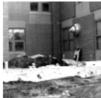
NW Footings - Stilwell
