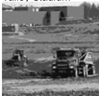
Hauling dirt - Valley Stadium
