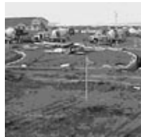
Footings Complete - Valley Stadium
