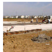
Concrete poured, north lot - Valley Stadium
