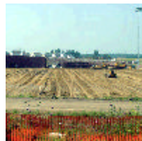
Field subgrading - Valley Stadium
