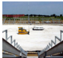
Grading - Valley Stadium
