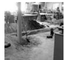
Shop Excavation - Stilwell
